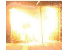
ARC FLASH INCIDENT
